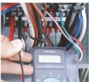
\* If the DC voltage between transmission terminal A, B of indoor unit is fluctuate within (-9V~+9V) then transmission from outdoor unit is normal
